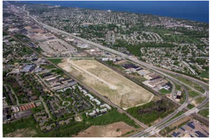
BLUESTONE INDUSTRIAL PARK
